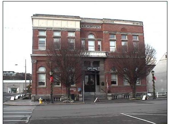
The 1892 Port Townsend City Hall is being renovated according to national green building standards.
